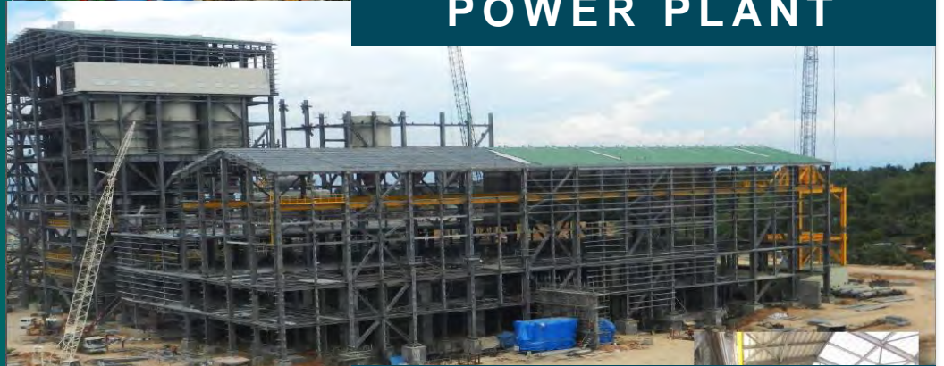
LIMAY 2X150MW POWER PLANT
